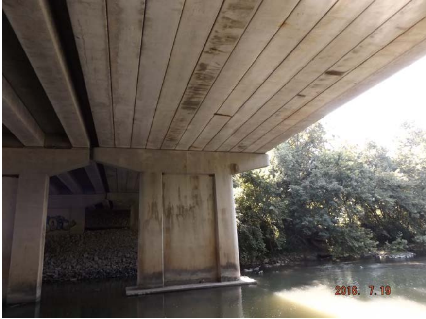
SUPER/SUB STRUCTURE - RIGHT
