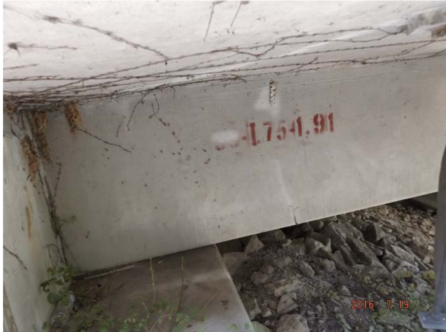
BRIDGE # - SPAN 1 - BEAM DD
