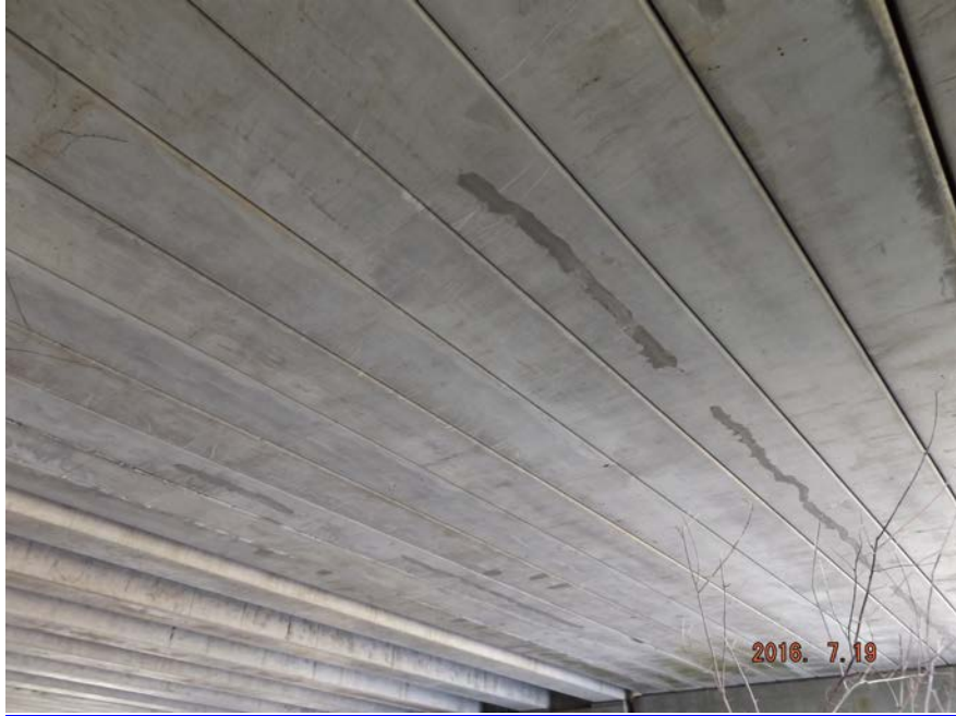
SPAN 3 - LEFT - CRACK REPAIRS
